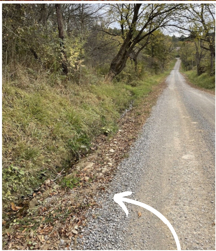
Before: Left hand side of the road and road ditch would blow out at every storm event.
