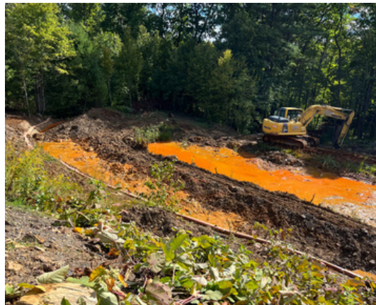
Right: Construction at the Clarion County Park AMD Treatment System.
